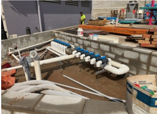
Manifold controls for Adventure Play area 05/10/2023
