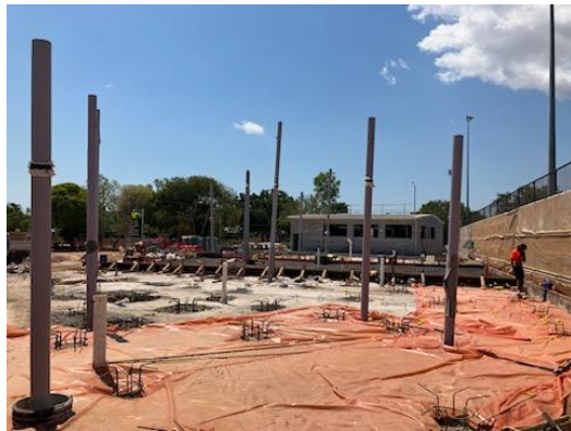
Ground structure and shade columns for adventure play area 06/09/23
