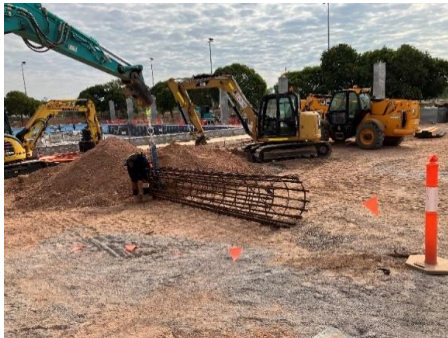
Preparing concrete piers south side of 50m pool 29/07/23
