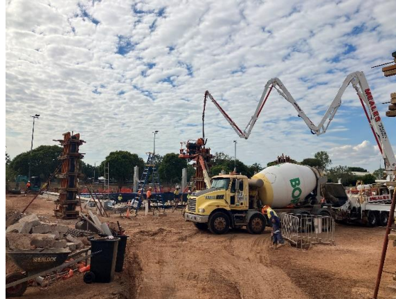
Pouring structure columns on north side of the pool 29/07/23
