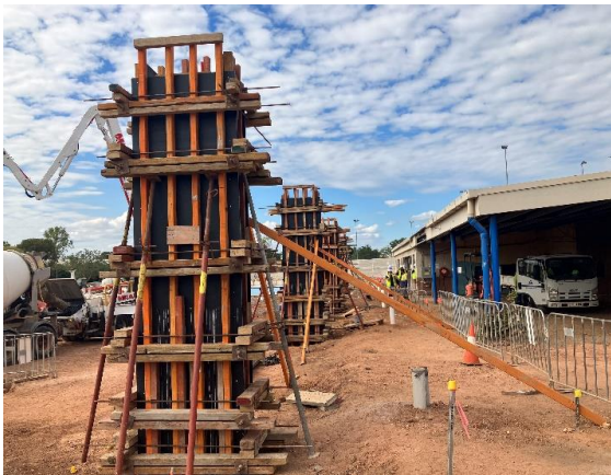
Pouring shade structure columns on south side of the complex 29/07/23
