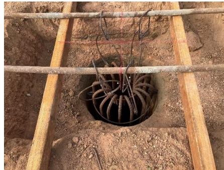
Pier steel supported on south side of 50m pool 29/07/23
