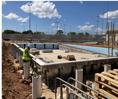
Program pool showing Myrtha gutters 06/06/23
