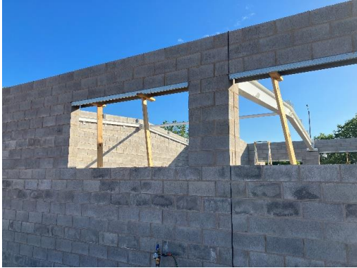
Plant Room Walls with Structural Steel Commenced 05/05/2023
