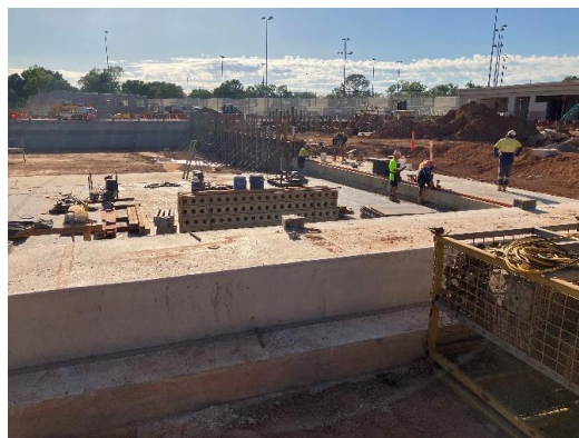
Right Side of 50m pool showing walls being readied for Myrtha installation 05/05/2023
