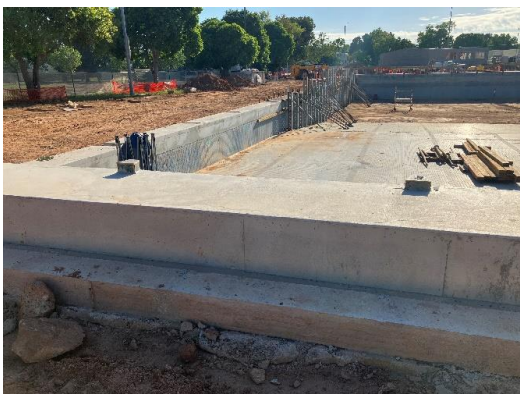
Left side of 50m pool showing walls ready to have Myrtha applied 05/05/2023
