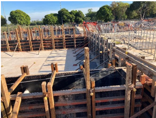
Program pool with walls formed ready for Myrtha 05/05/2023
