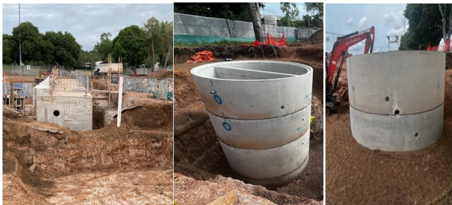
Balance tank and sewer pump station
