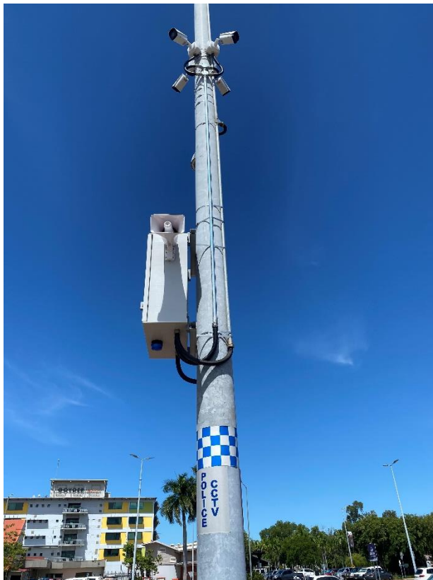
Police CCTV Pole with cameras and speakers
