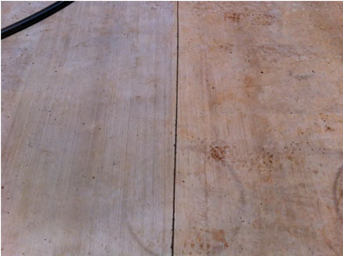
Image 1: Left panel – citric acid cleaner, right panel detergent and pressure wash
